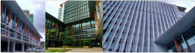
Fig. 4. Multiple external shading system of Menara PjH.
