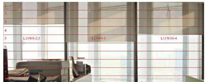
Fig. 6. Estimation of blind position for occlusion index
