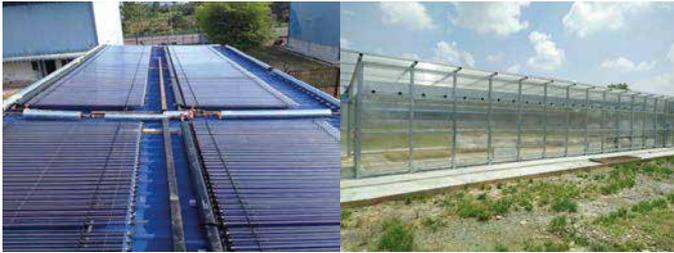
Fig. 2: Evacuated tube (left) and the drying chamber (right) from short distance.
