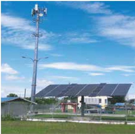
Figure 1. Photograph of Standalone Double Axis Solar Tracking System with Maximum Light Detection (MLD)
