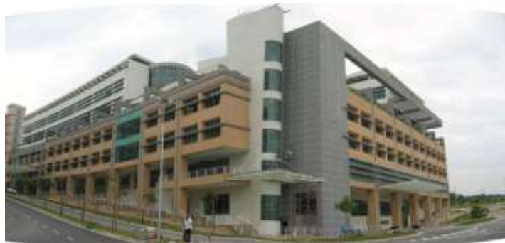
Ministry of Energy, Green Technology and Water, Putrajaya, Malaysia Year of completion: 2004
