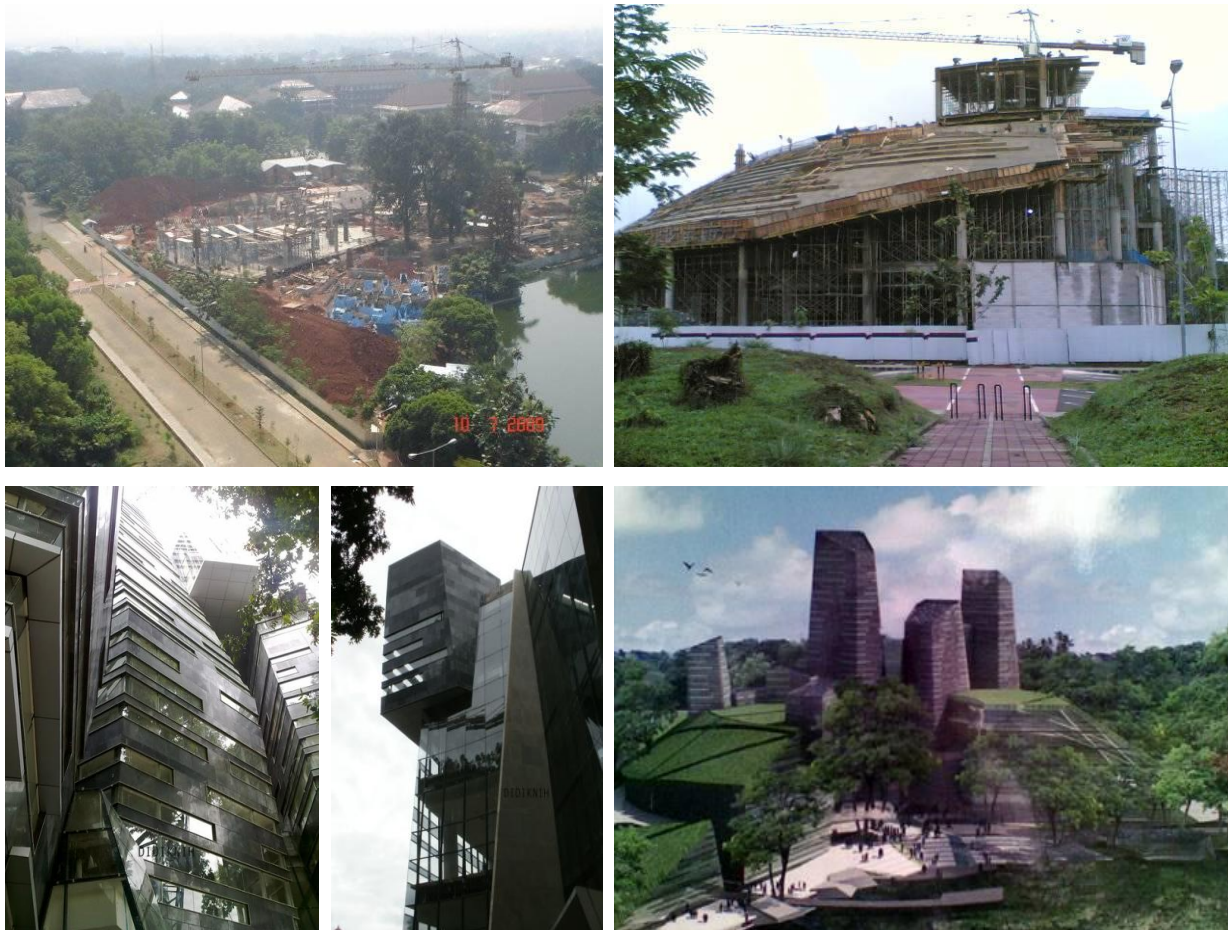
Figure 3,4,5 & 6 : Central Library, University of Indonesia (source : Denton Corker Marshall , 2009)
