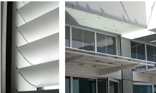
FIGURE 4.4 | EMBEDDED BLINDS IN DOUBLE GLAZING WITH EXTERNAL LIGHT SHELVES (GEO BUILDING, MALAYSIA)
