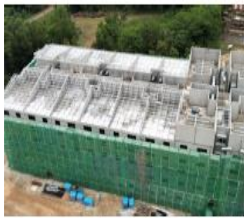
Form a Completed Unit
