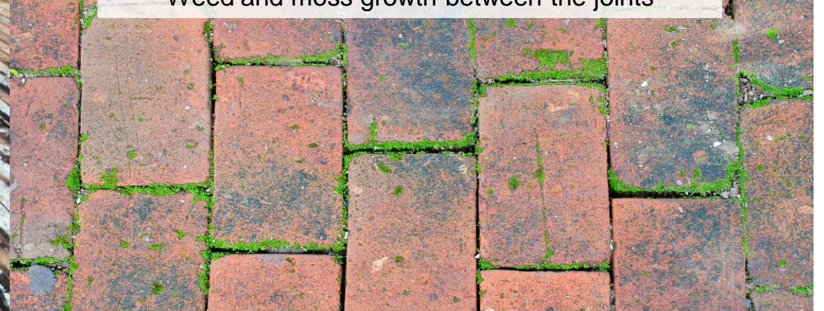
Weed and moss growth between the joints
