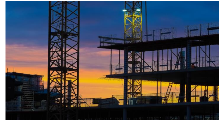
Allows construction to continue through the night
