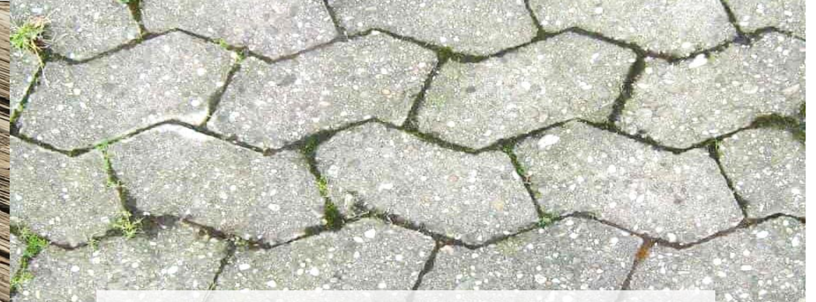
Weed and moss growth between the joints
