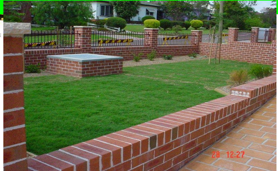
Above ground OSD system for a townhouse in Holroyd, Australia.
