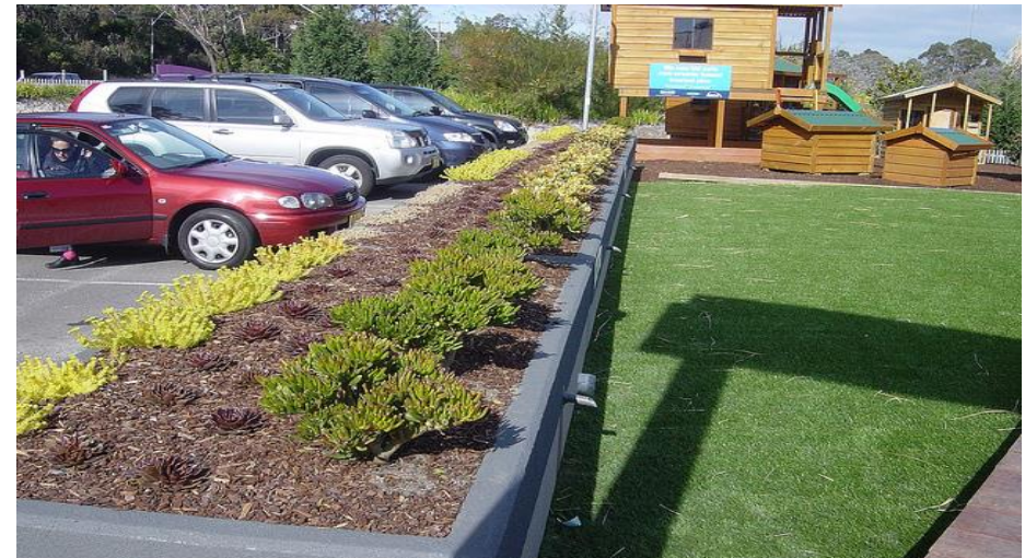
OSD Landscape Tank in public area.
